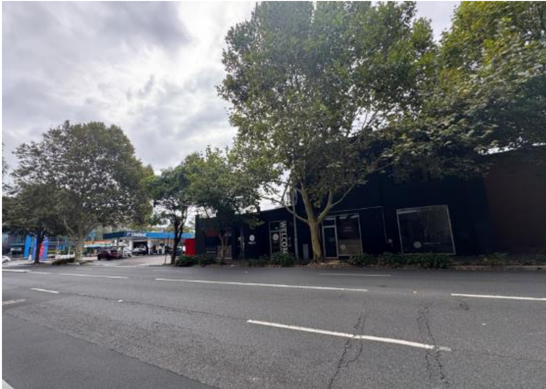
Figure 8: Existing developments 941-953 and 937-939 Bourke Street to the south of the site
