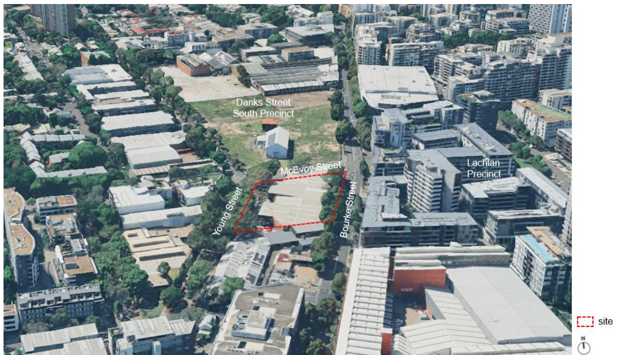
Figure 2: Site and surrounds (Source: Google Earth)
