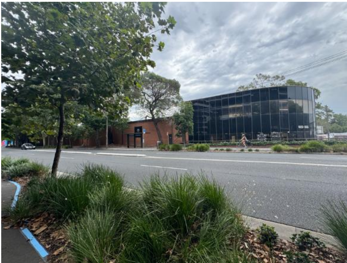
Figure 4: Site viewed from Bourke Street
