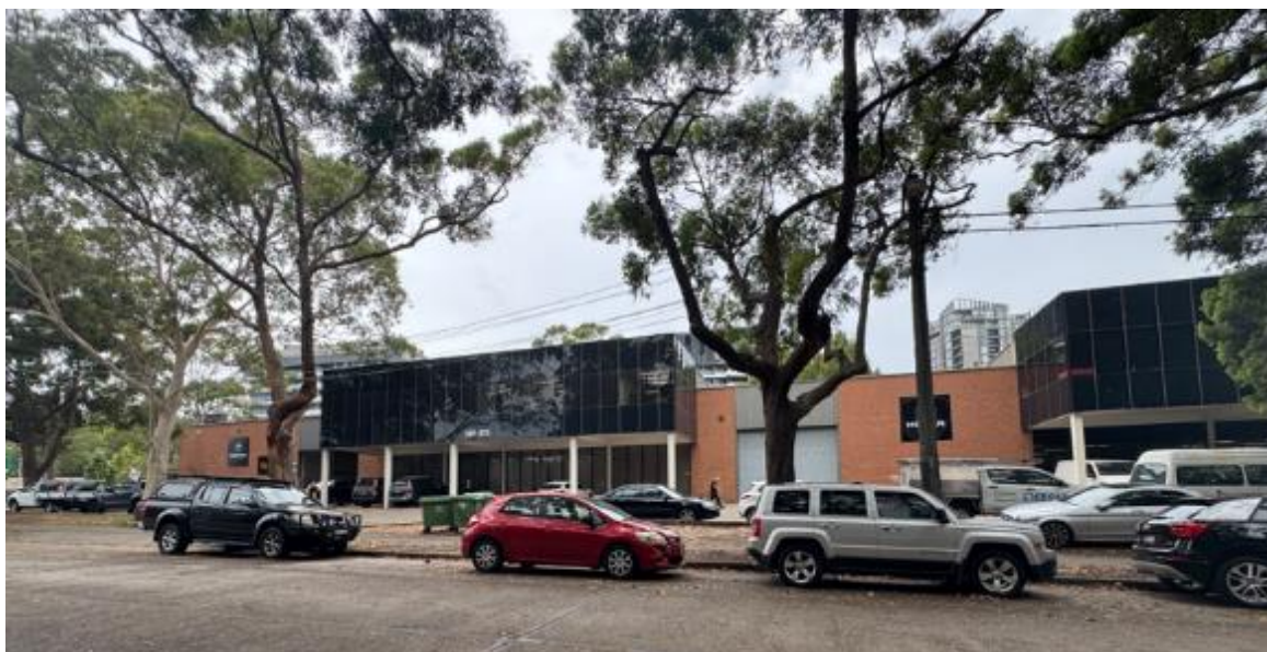
Figure 6: Site viewed from Young Street
