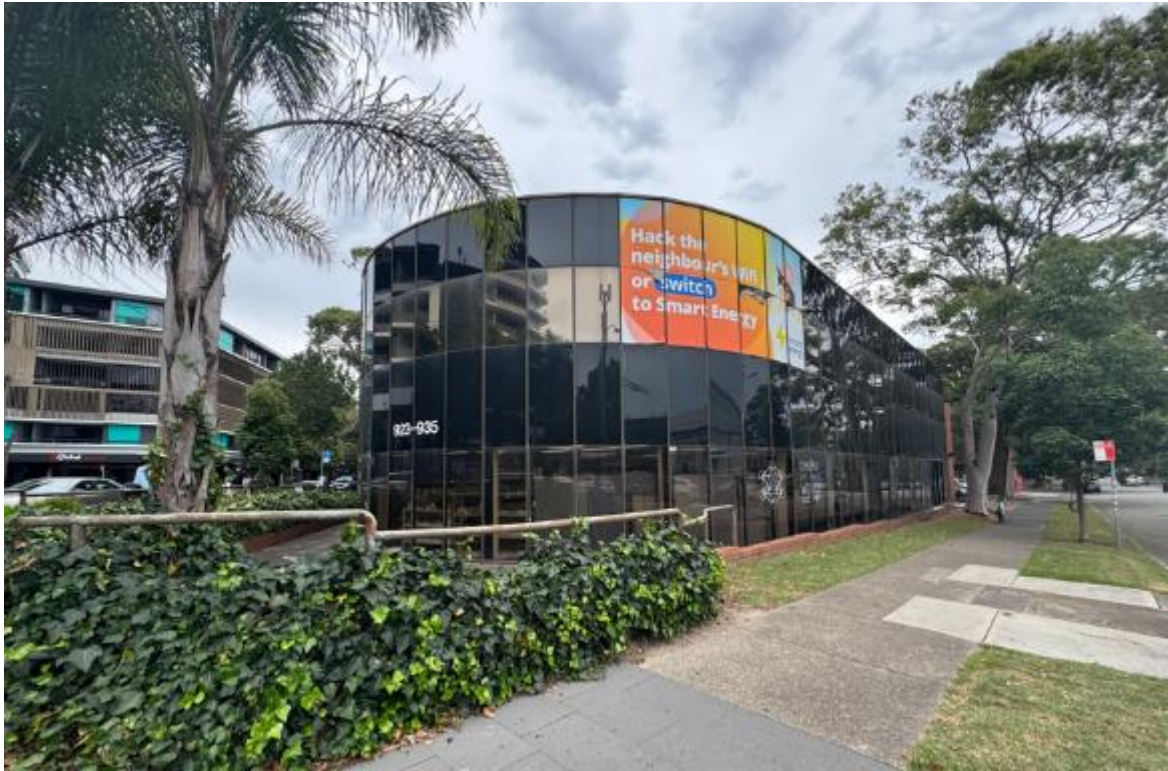
Figure 3: Site viewed from McEvoy Street
