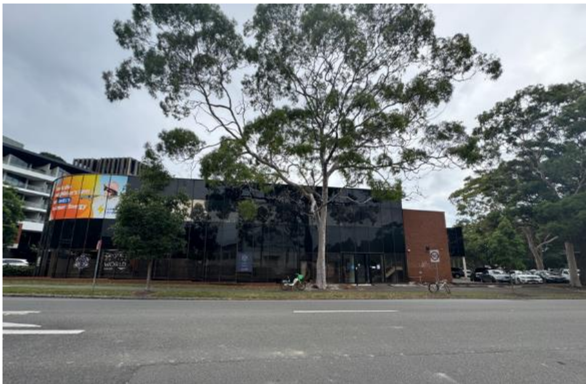
Figure 5: Site viewed from McEvoy Street
